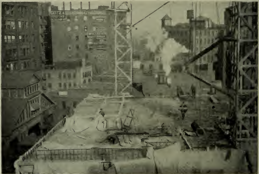
FIG. 6. PROTECTING CONCRETE WITH TARPULINS IN WINTER.
